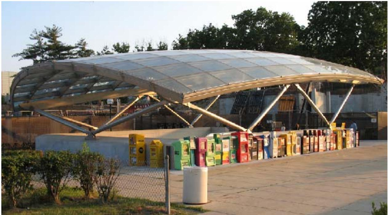
Figure 8: UNS S32003 alloy used in piping for structure support. Canopy from the Medical Center Metro Station in Bethesda, MD.
