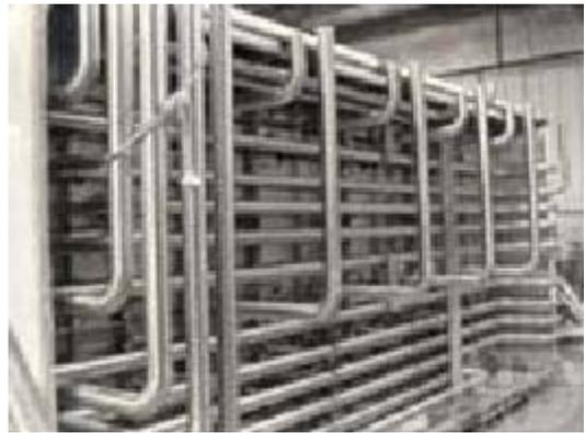
Figure 6: In-Plant Piping of UNS S20153 alloy
